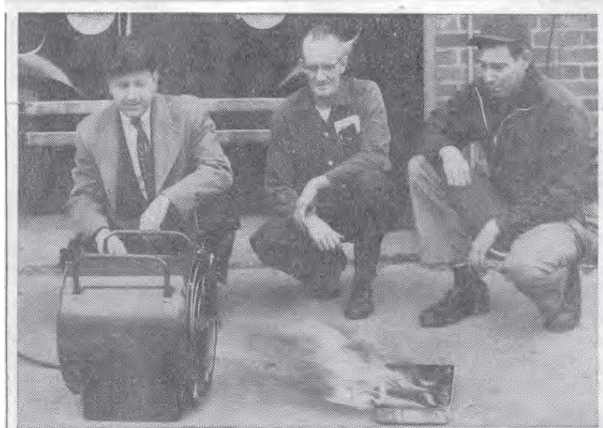
JUST FANNING THE BREEZE—New Hartford fire officials watch test run on department's new smoke ejector—first in use in Oneida County. Ejector is utilized in after-fire mopping up operations. Three-blade fan, making 1,725 revolutions a minute, dispels smoke, gas and other fumes. Tank attachment contains deodorizer which is blown over area to kill unpleasant odors. One-third horsepower motor can be operated by portable generator. Observing "dry run," from left, are Assistant Chief Harold Lewis, fireman Bert Andrews, and Chief Edward Roman Jr.
